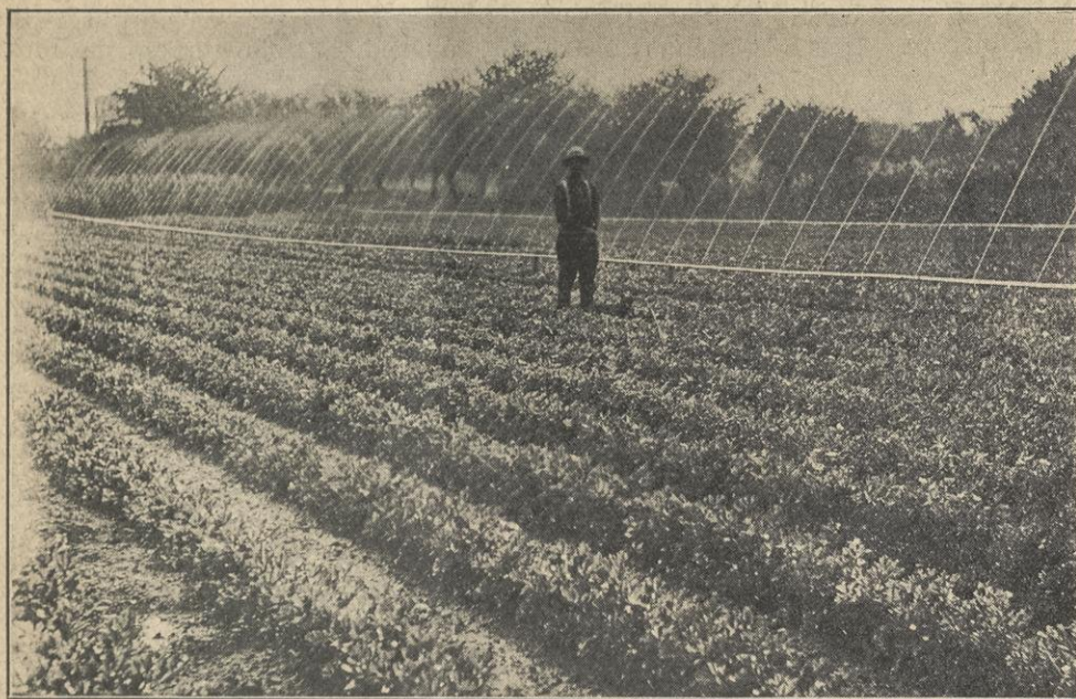
The Skinner Sprinkler System as used in his celery patch by Mr. Buck, of Freeman, Ont. The pipes can be turned to throw water to either side.
