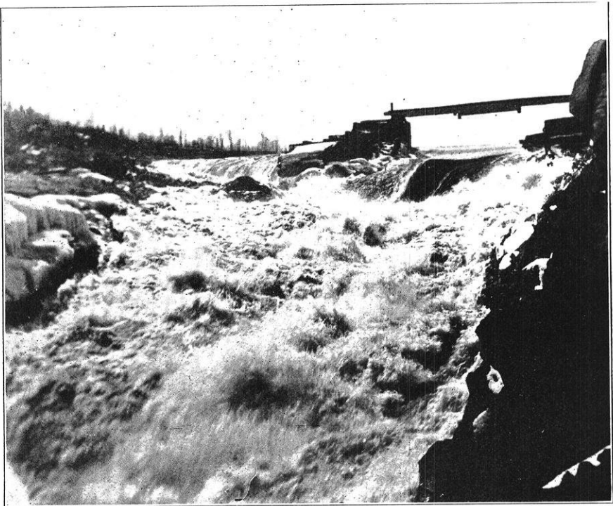
Upper Quinnesec Falls, Near Iron Mountain, Mich., Menominee River, 54 feet head improved.
