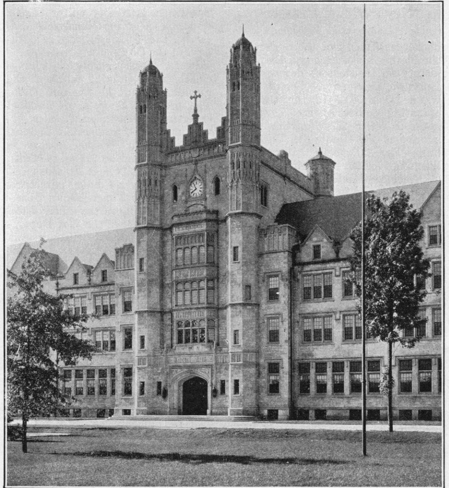
Liberal Arts Building, Marygrove College, Detroit, Mich. D. A. Bohlen & Son, Architects. W. E. Wood Co., Builders. Variegated Indiana Limestone Random Ashlar.
