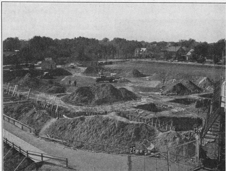
DIGGING THE FOUNDATION
