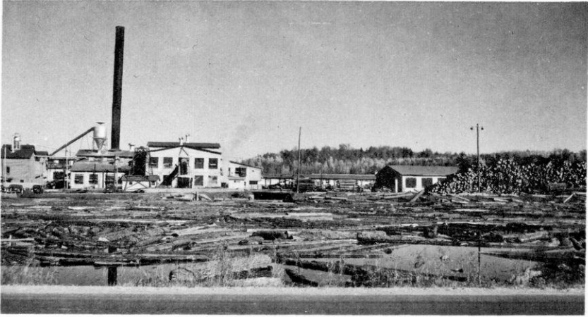
Figure 7. A view of the lumber mill at Neopit.
