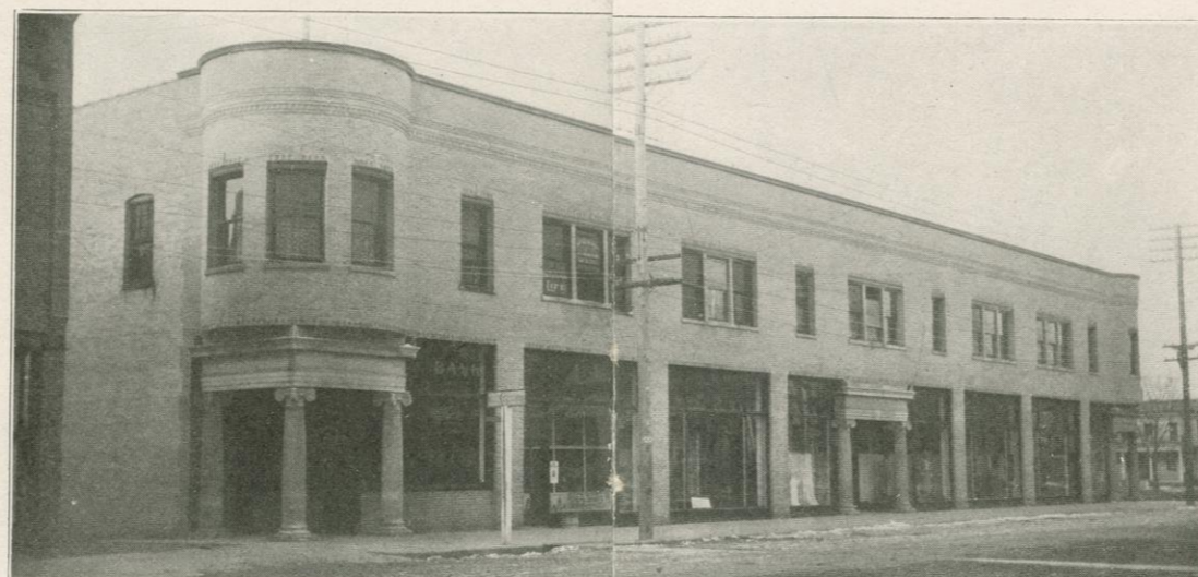
The Grange Block
