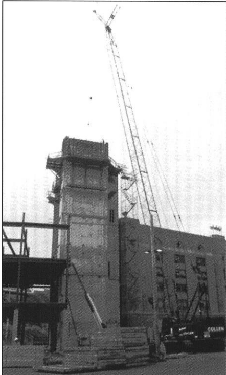
A crane moves 42,950 pound concrete panels.
