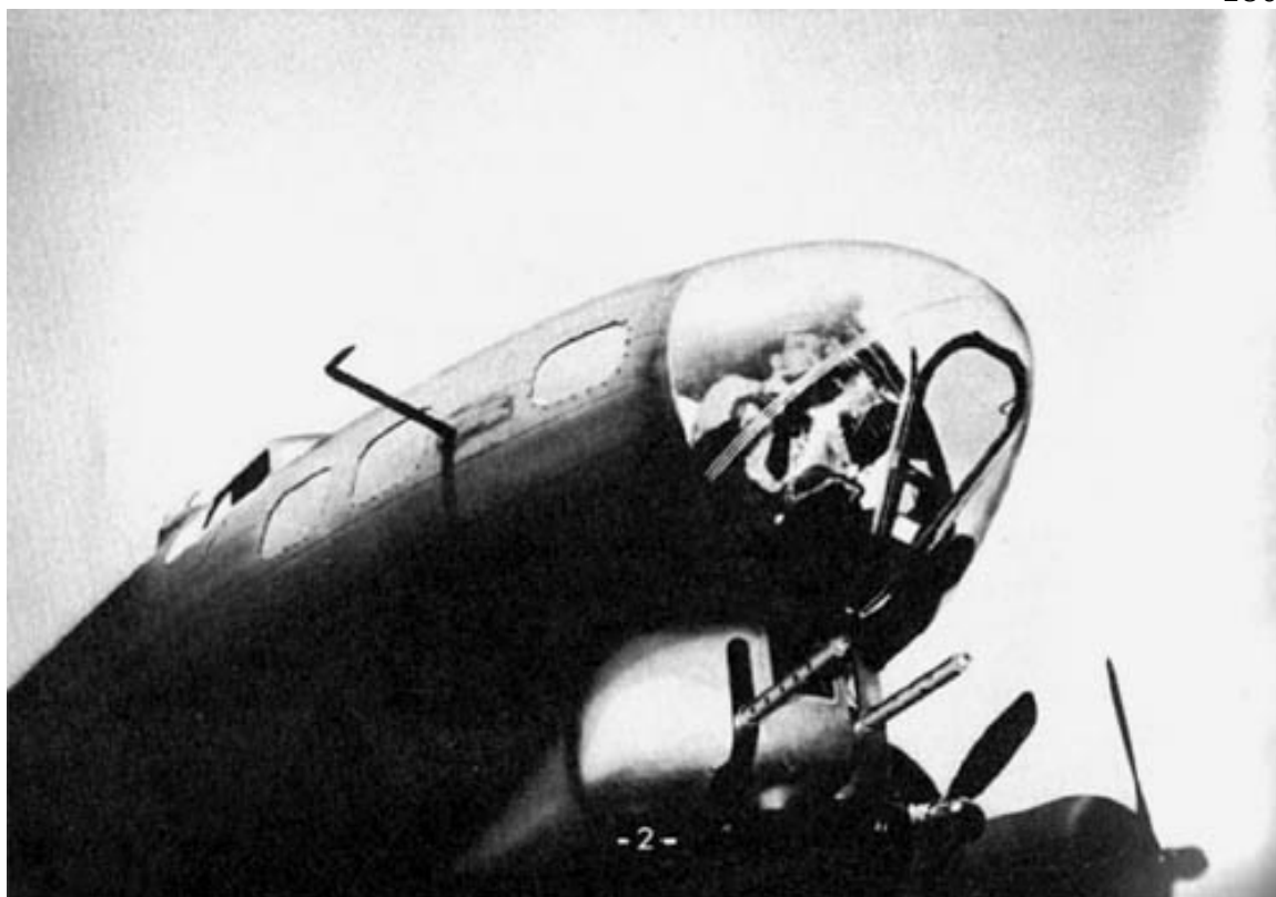
FIGURE 6: Plexiglas turret on a B-17 bomber plan, Circa 1944. Image from: http://www.lonesentry.com/blog/bendix-chin-turret.html
