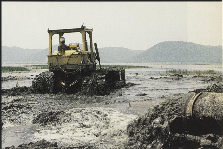
Skilled heavy equipment operators pile sand and sculpt islands. Their designs work with nature so upstream portions are protected and downstream sides flood as the river rises.
