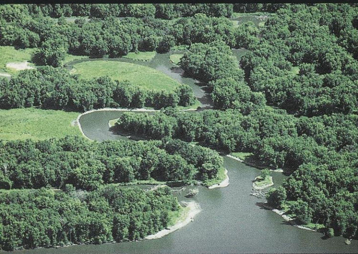
Better habitat through engineering — At Bertom and McCartney lakes, a 1,500-foot, rock-lined channel connects backwater pools, oxygenates water and provides winter habitat for fish.
