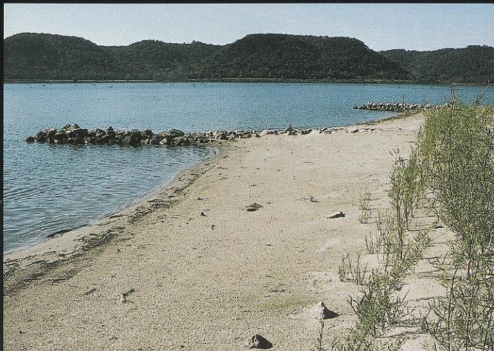
Rock groins trap sand and silt carried in the Mississippi's turbid water. As the current slows, solids form a beach and stabilize the islands.
