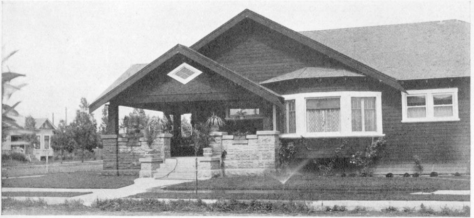
A CLAPBOARD HOUSE WITH PORCH FOUNDATION AND CHIMNEY OF CREAM SANDSTONE AND TRIMMING OF CREAM WHITE: COST $3,000.
