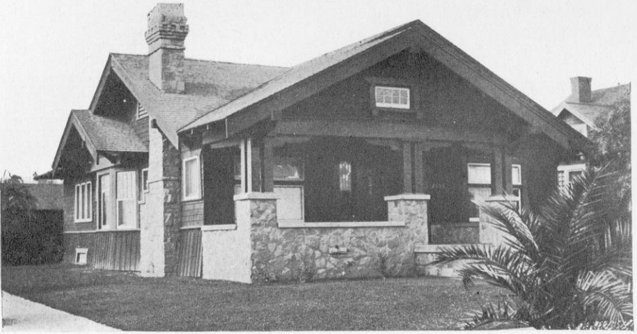
BUNGLOW BUILT FOR $3,300: INTERESTING SIMPLE WOOD CONSTRUCTION, WITH FOUNDATION, PORCH AND PORCH PARAPET OF WHITE LIMESTONE.
