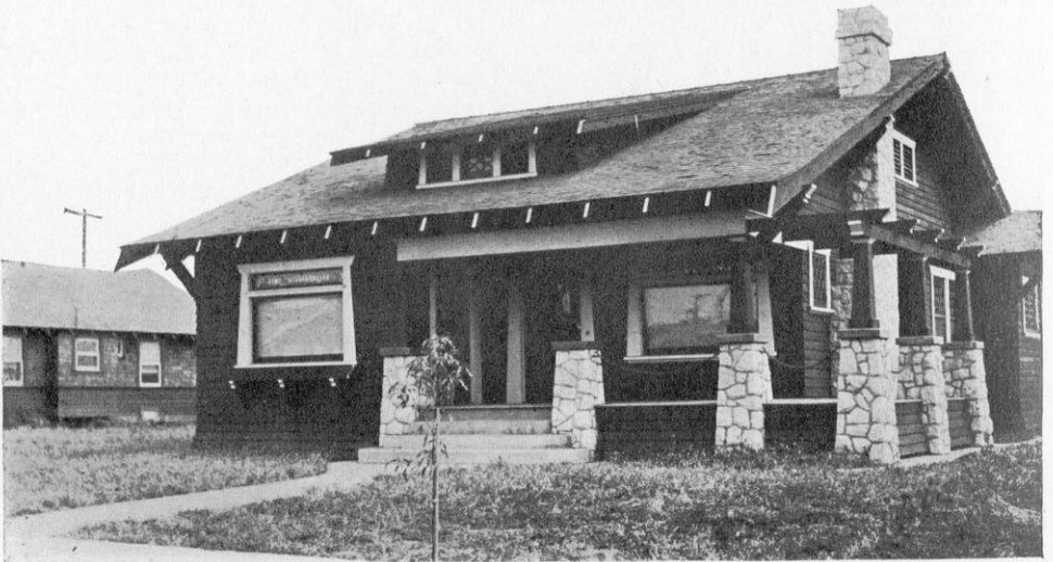
$2,800 CALIFORNIA COTTAGE WITH UNUSUAL WINDOW ARRANGEMENT IN THE ROOF AND WITH PICTURESQUE PORCH PILLARS AND CHIMNEY OF LIMESTONE.
