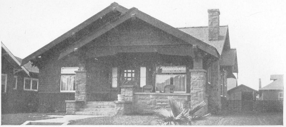
A SMALL CALIFORNIA BUNGALOW COSTING $3,200, SHOWING THE USE OF RED SANDSTONE FOR PORCH PILLARS, PORCH FOUNDATION AND CHIMNEY.
