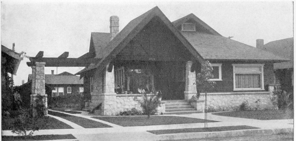
BUNGALOW COSTING $3,800, WITH WHITE LIMESTONE USED FOR FOUNDATION, PORCH AND PERGOLA: JAPANESE EFFECT IN WOODWORK.
