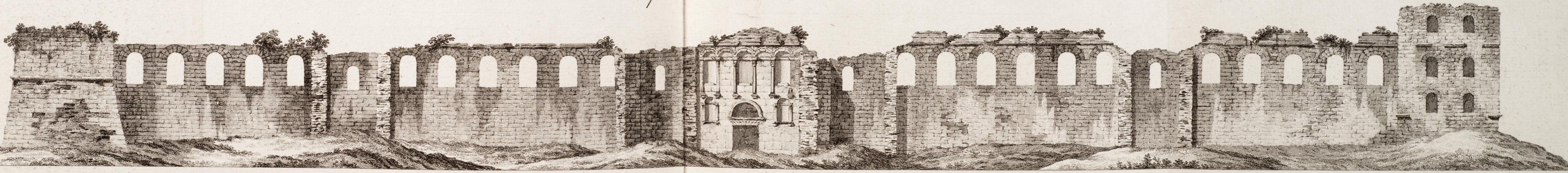
Elevation of the Same Wall as it now Remains
