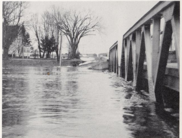
1961 - Flood at Hogarty Bridge Highway 52
