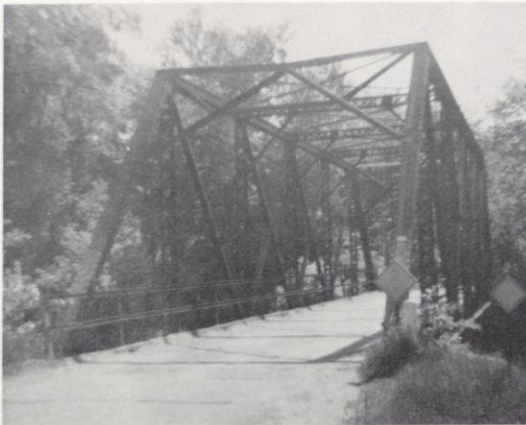
Former bridge on Highway G.
