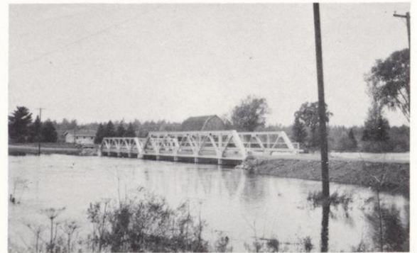
Newly constructed Eau Claire River Bridge 1959
