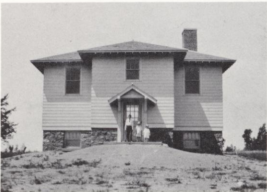
Newly constructed Fallow School in about 1928.
