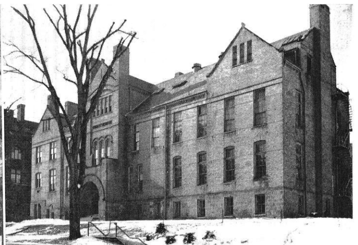
The Aged Chemical Engineering Building
