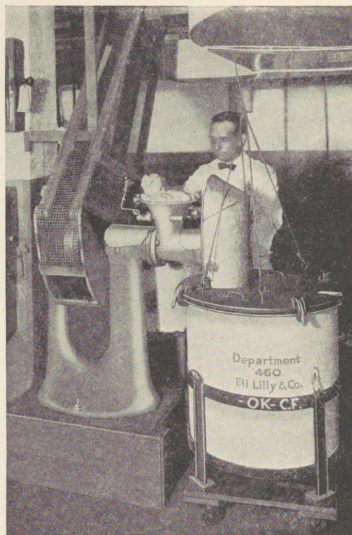
Before the alcoholic extraction the pancreas glands are run through grinders.
