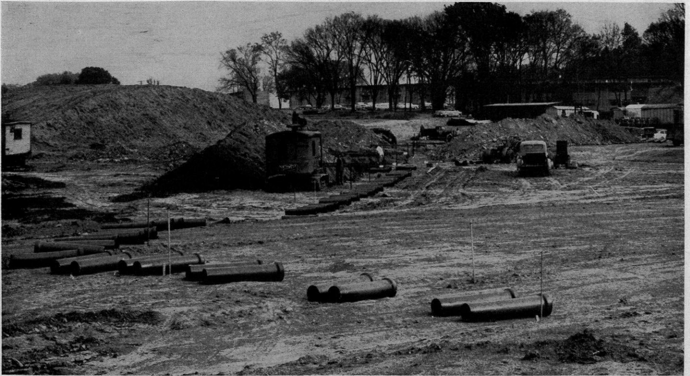
EAGLE HEIGHTS APARTMENT CONSTRUCTION
