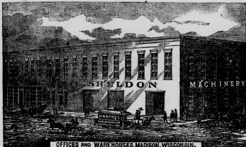
OFFICES AND WAREHOUSES, MADISON, WISCONSIN.
