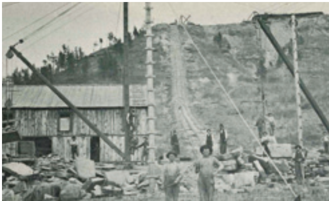
A tramway operated by the Goodyear Lumber Company moved quarried stone down the south slope of Saddle Mound.
