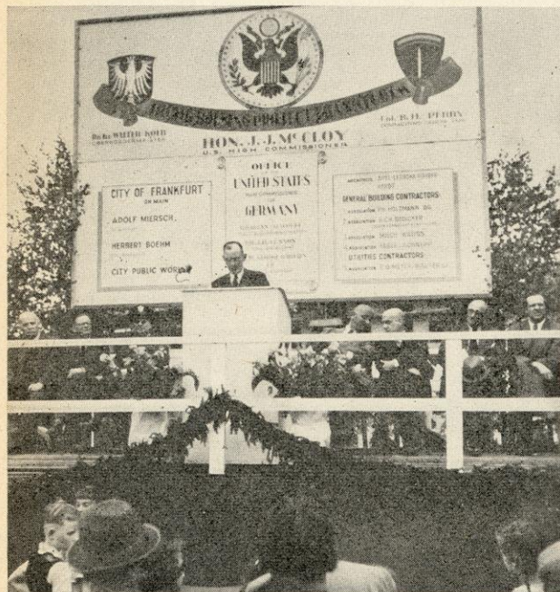
Delivering the principal address at the "Richtfest"—traditional German roof-raising celebration—was Maj. Gen. George P. Hays, at the halfway construction mark in the HICOG housing project in Frankfurt. The Deputy US High Commissioner shared the rostrum with Frankfurt's Mayor Walter Kolb, Glenn G. Wolfe, director, Office of Administration, and other US and German officials. (PRD HICOG photo)
