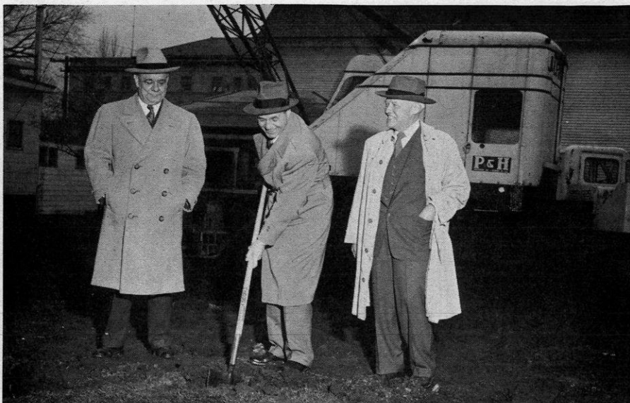
GOV. WALTER Kohler was on hand to scoop out the first shovel full of dirt when work was begun this spring on the intern-resident dormitory. The $710,000 structure will house 80 interns and resident doctors from Wisconsin General hospital. Shown with Kohler are Regent A. Matt Werner, left, and Dr. Harold Coon, superintendent of Wisconsin General, right.
