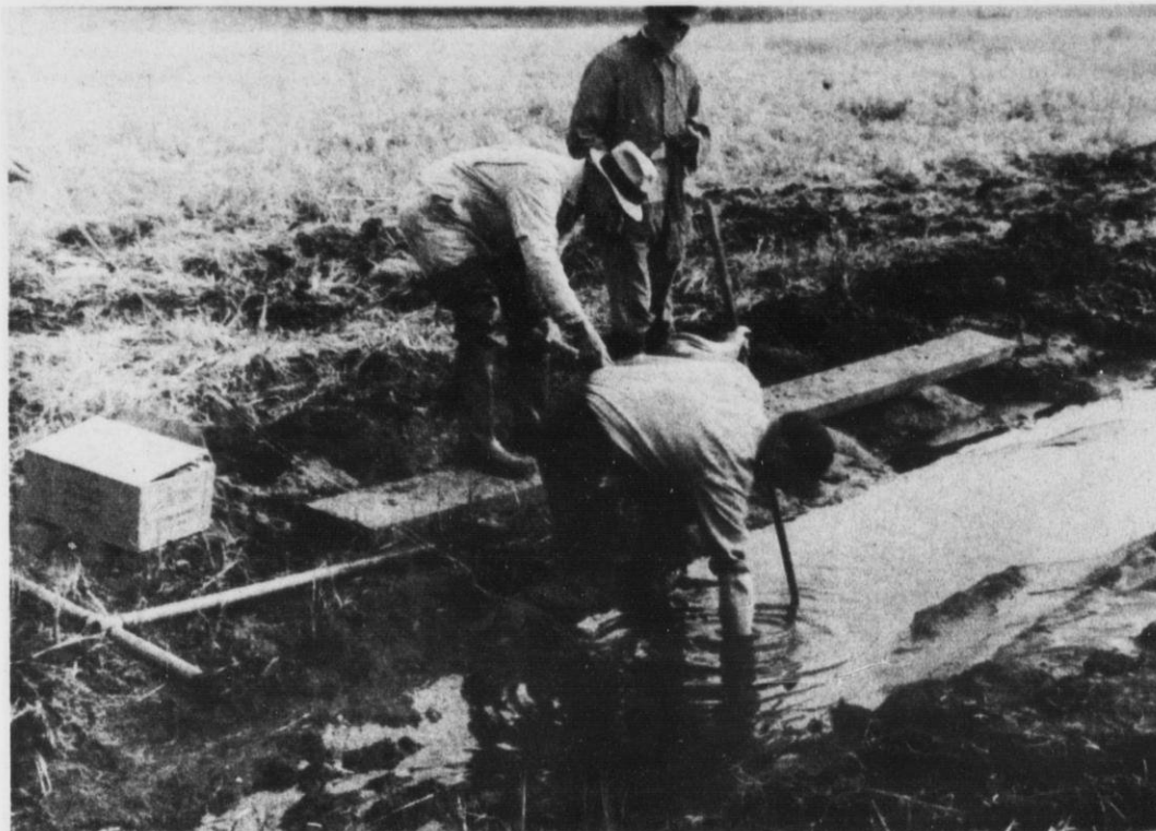
Ditching is difficult, if not impossible, in many areas where the surface soil remains too wet to enable a tractor to operate. Ditching with dynamite is a solution on many farms. B. F. Gustafson is shown loading, with Elmer Miller and Andrew Schroedel observing on the Gross Brothers farm, Sigel town.
