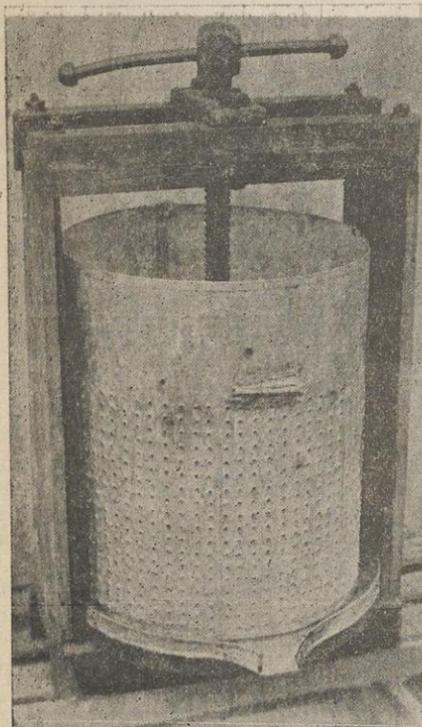
size of the can go in the top for the screw to act on, made of 1 in. hardwood, spring made of 4 x 1 in. battens, 12 in. long, with a piece  $\frac{1}{2}$  x 1 in. across, under each end of the first, and one under the centre
