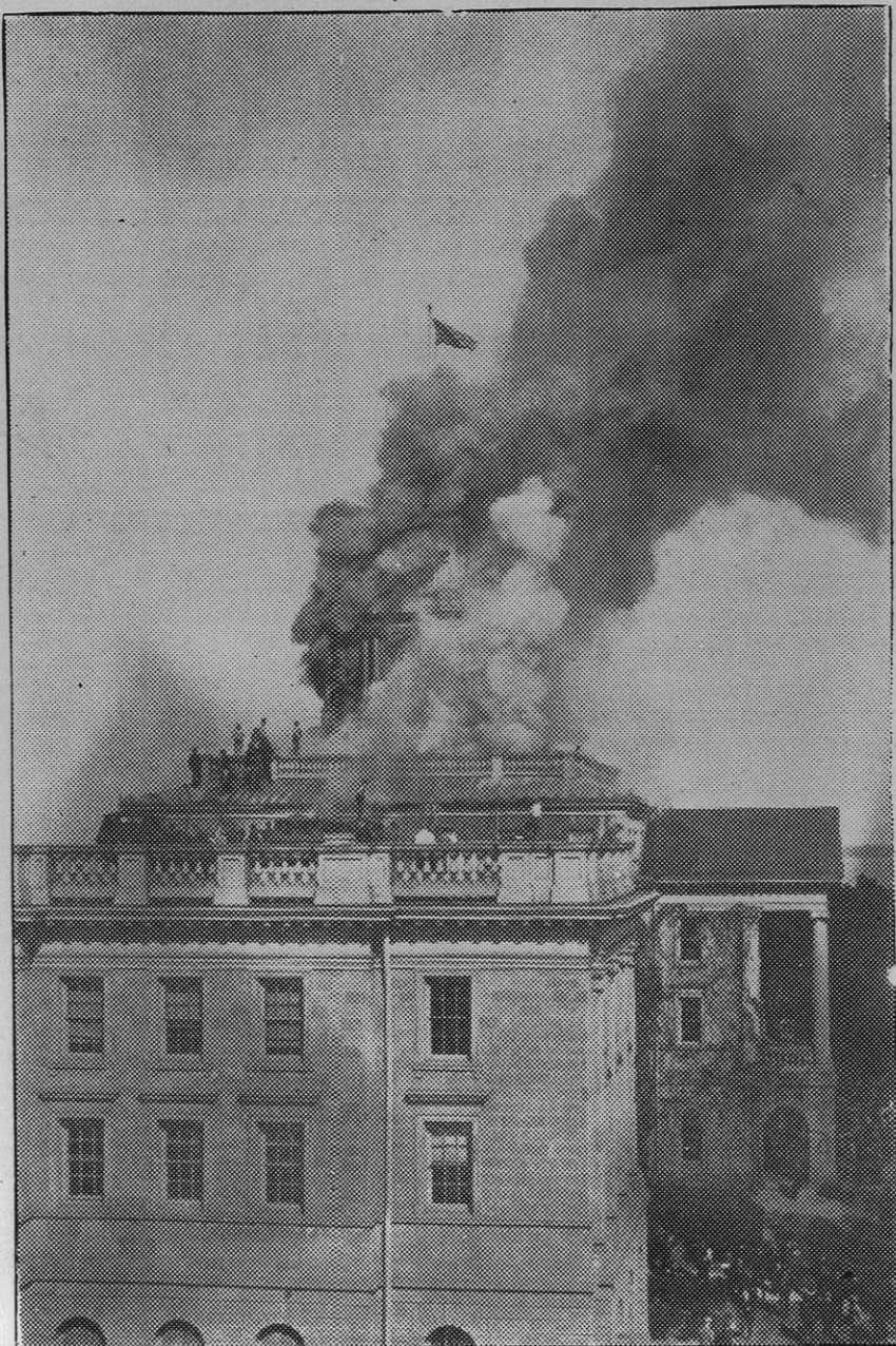
MAIN HALL FIRE
