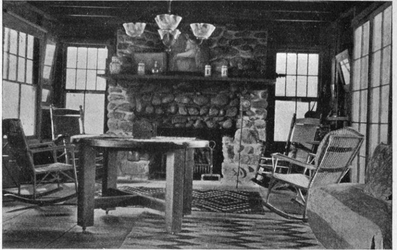
FIELD STONE CHIMNEYPIECE FOR COUNTRY HOME.
