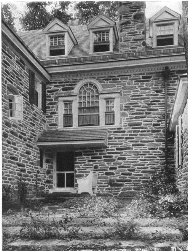
FIGURE EIGHT : DETAIL OF MR. BROWN'S HOUSE : THE STONEWORK IN THIS HOUSE IS RATHER FORMAL, AL- MOST PRIM : THE STONE IS SPLIT AND THE ENDS ROUGHLY SQUARED SO THAT IT CAN BE LAID IN COMPARATIVELY EVEN COURSES AND THE STONES ARE OF NEARLY EQUAL SIZES THROUGHOUT : THIS METHOD OF LAYING UP STONES IS SEEN VERY OFTEN IN THE OLD DUTCH HOUSES IN REMOTE PARTS OF NEW JERSEY.
