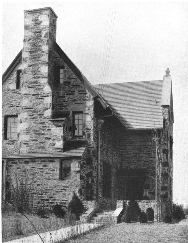
FIGURE FOUR : DETAIL OF A FIELD-STONE HOUSE DE- SIGNED BY MELLOR AND MEIGS : THE USE OF LARGE STONES AS "QUINS" AT THE COR- NERS OF WALLS AND CHIMNEYS IS ESSENTIALLY STRUCTURAL AND MOST CRAFTSMAN- LIKE. THE LOOK OF SOLIDITY AND DURABILITY WHICH IS GIVEN BY THIS METHOD OF TREATING FIELD STONE IS ONE WHICH REN- DERS THE MA- TERIAL ESPE- CIALLY SUITABLE TO LARGE COUNTRY HOUSES OR TO RURAL CHURCHES : THIS TREATMENT COULD BE DUPLICATED IN A GARDEN WALL WITH A MOST INTEREST- ING RESULT.
