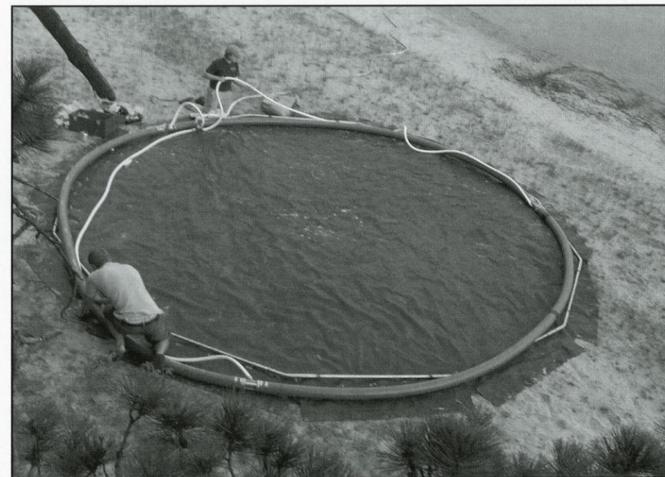
The GELI creates a column of warm water, raising temperatures to levels uninhabitable by invasive smelt.
