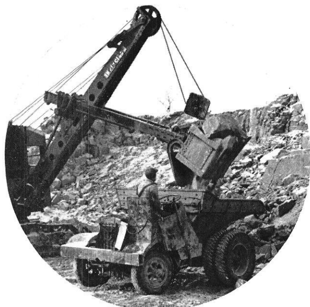
Loading a Dump Truck
