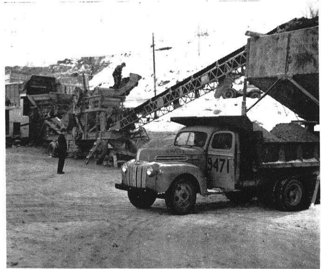
Loading Gravel, Which Is Plentiful Along the Highway Route
