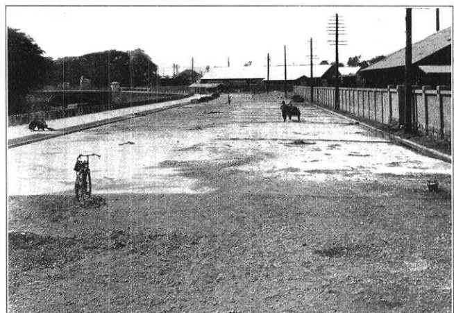
Same street after completion, widened from 32 to 90 feet
