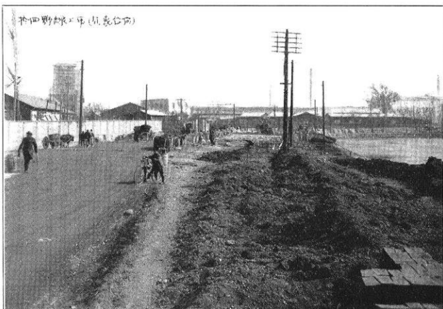
Widening of street by filling in of Canal
