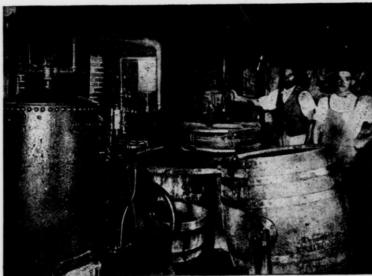
FIG. 8.—Interior of Five Corners factory, showing a cheese in the press and the means of adjusting the pressure. The small engine and churn are for making whey butter.
