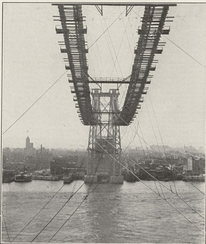
VIEW BENEATH NEW EAST RIVER BRIDGE DURING CONSTRUCTION OF WIRE CABLES.
