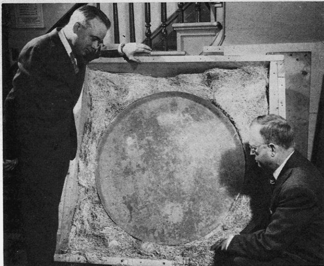
THE 600-POUND disc of glass shown above will some-day mirror the heavens. Purchased by the University with Alumni Research foundation funds, it is the first step toward a new 36-inch reflecting telescope to supplement the 71-year-old, 15½-inch reflector being used in the University's Washburn observatory. Shown inspecting the disc are University astronomers A. E. Whitford and C. M. Huffer (left). They estimate that it will take at least four months to grind the disc into a concave mirror.
