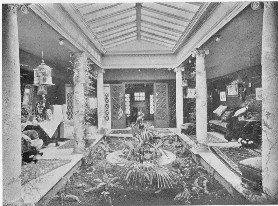
VIEW OF THE PERGOLA ROOF GARDEN. THE LUMBER IS PINE LEFT ROUGH AND STAINED DULL GREEN. ONE END OF THE PATIO, SHOWING GLASS ROOF WHICH IS LEFT OPEN IN SUMMER.
