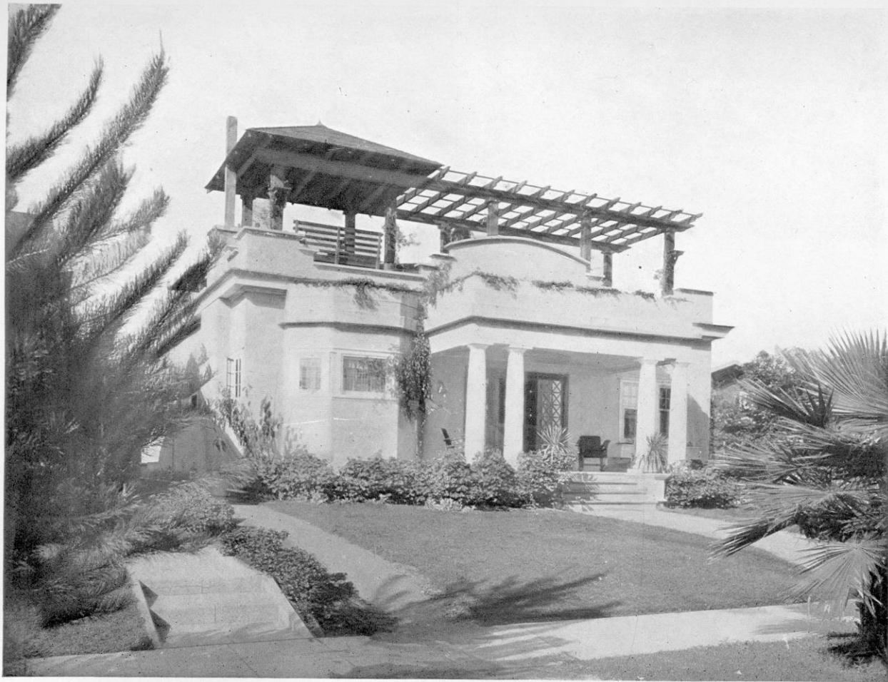
A PASADENA PLASTER HOUSE IN MISSION STYLE, WITH ROOF GARDEN AND SPANISH PATIO.
