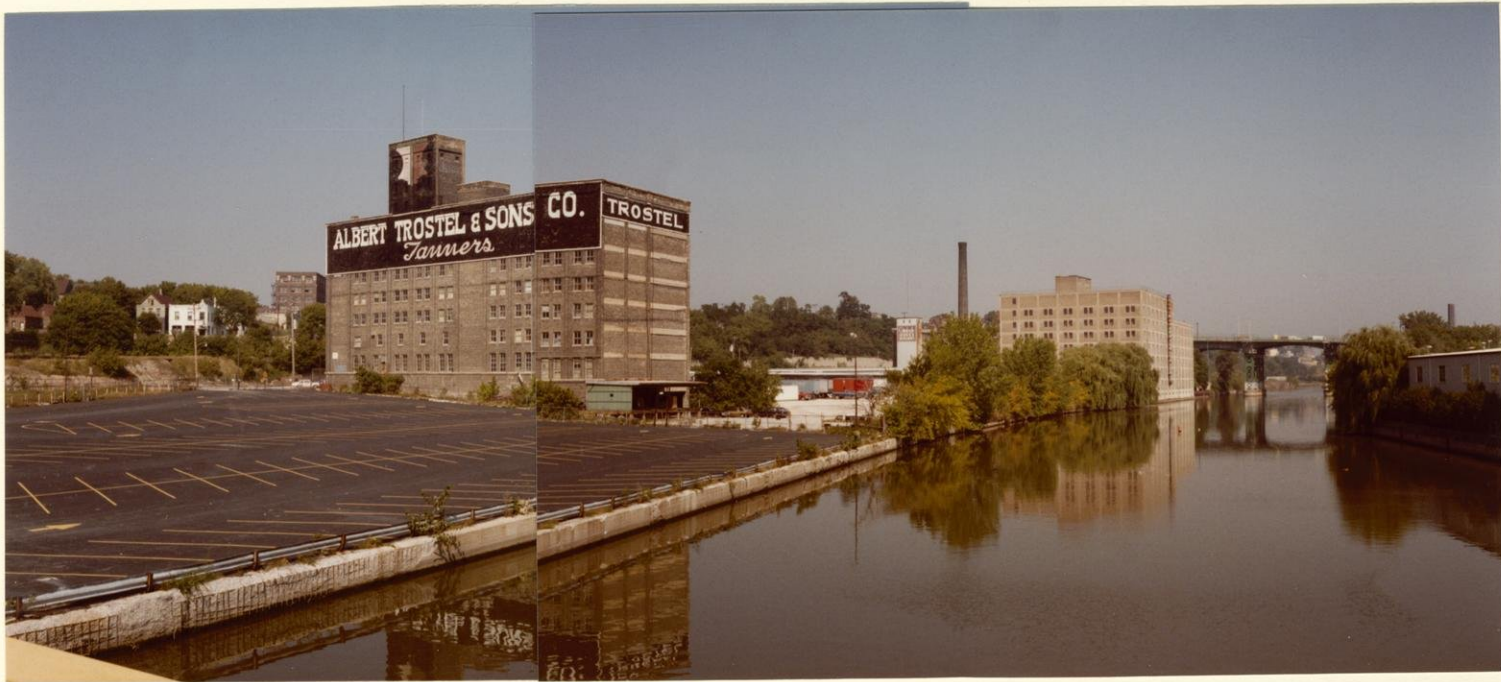
Trostel Site from Pleasant Street Bridge
