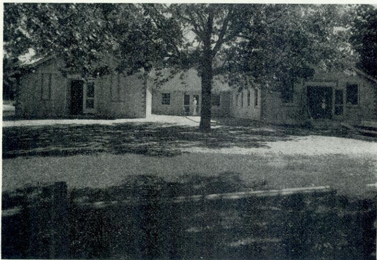
Mess hall and kitchen, Camp Williams, completed late in 1941.
