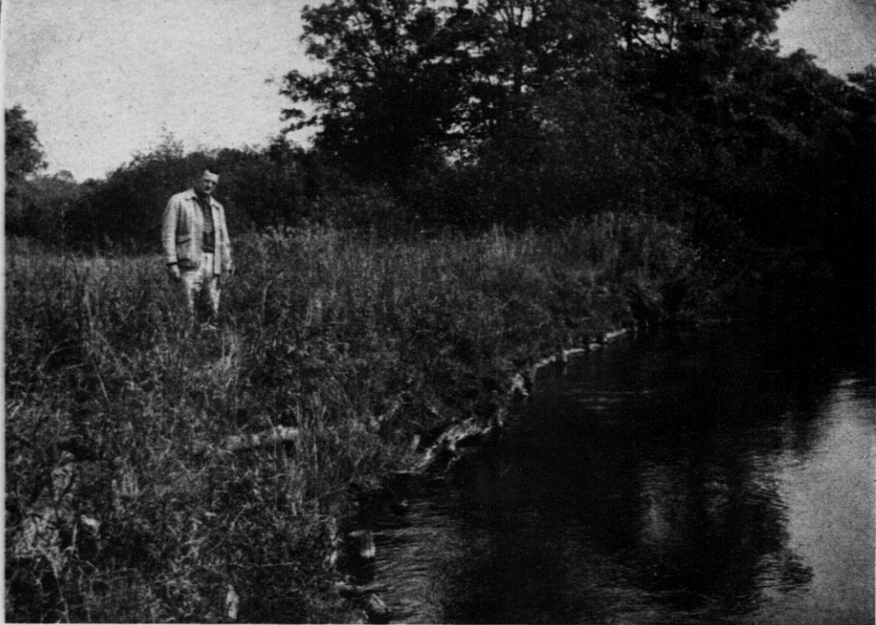
Protected stream bank one year after improvement. The bank cover is growing back.
