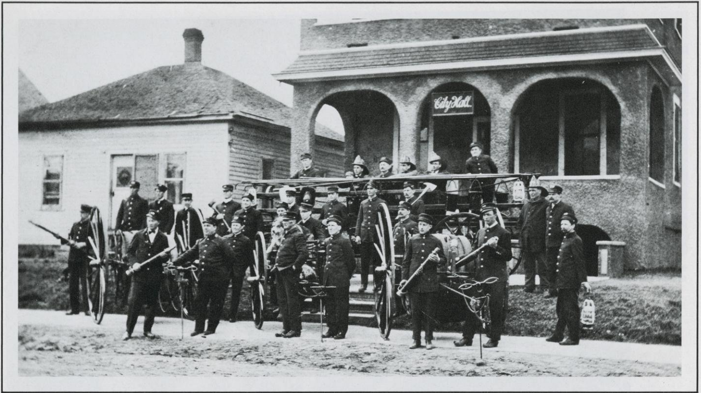
The Ladysmith Fire Dept. assembled in front of city hall for this picture sometime after World War I. The department had three hose carts and a pumper (which is mostly hidden). The dog on the center hose cart may have been the mascot. This equipment seemed antiquated when the department got its first truck in the late 1920s. The city remodeled the 1897 school house into city hall. The fire station was to the east of it.
