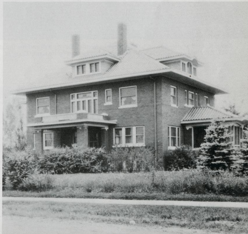
This view shows the north side of the N. J. Smith house in Ladysmith. The portico was wide enough to accommodate an automobile. The front porch is visible on the west side of the home. The structure was built at a cost of about $60,000.
