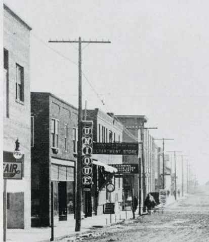
The Unique Theatre was new when this picture was taken in about 1914. The theatre sign was removed from the old building (now Pla-Mor Lanes) and attached to a telephone pole in front of the building. A marquee was later built. The Fair Store, operated by J. Kaufman, was north of the theatre. The Unique was destroyed by fire in 1951.
