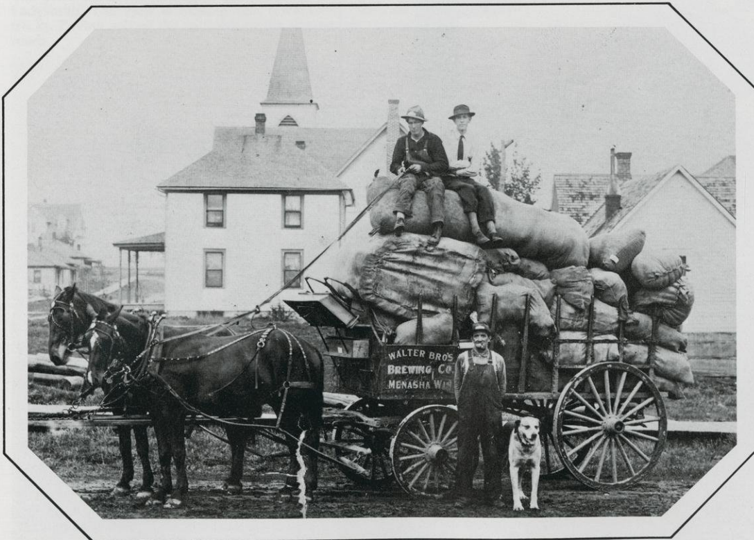
Although the writing on the side of the wagon refers to Menasha, this picture of a loaded wagon was taken in Ladysmith. The view looks north from Miner Avenue toward what was then St. Paul's Lutheran Church (now the Baptist Church). The house with the four windows was the parsonage. The operator of this dry line is not identified on the picture.
