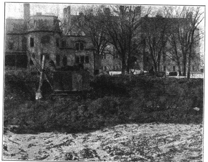
The "Diggings" for the Memorial Union is nearly completed
