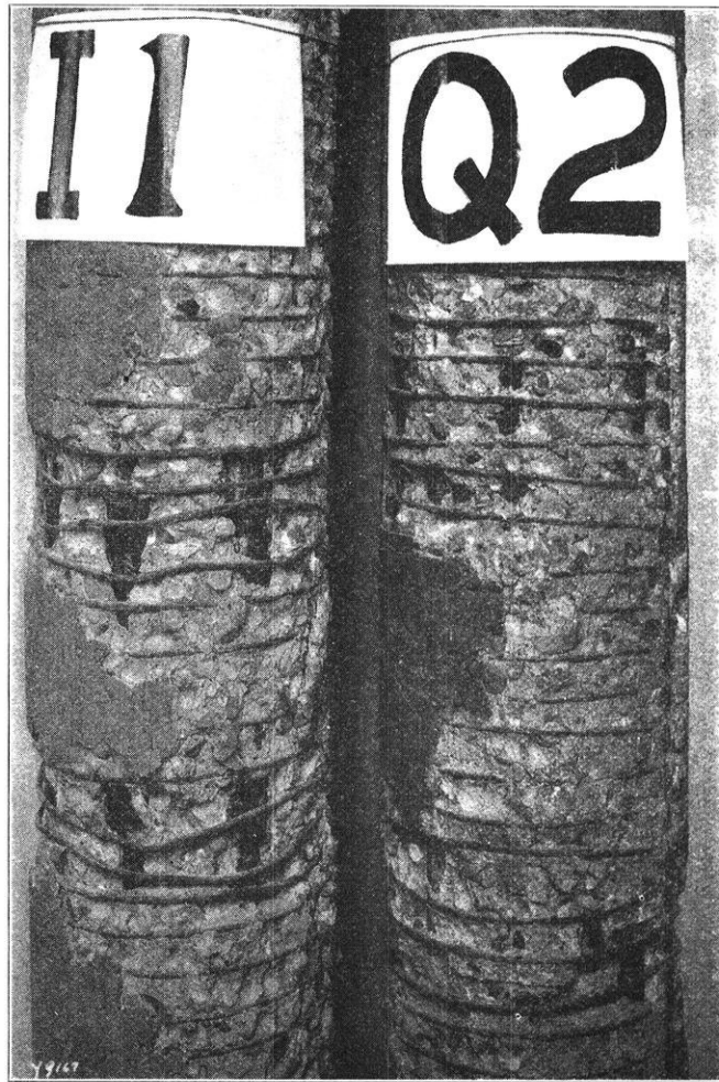
FIG. 4. Tested columns with splice rods exposed.
