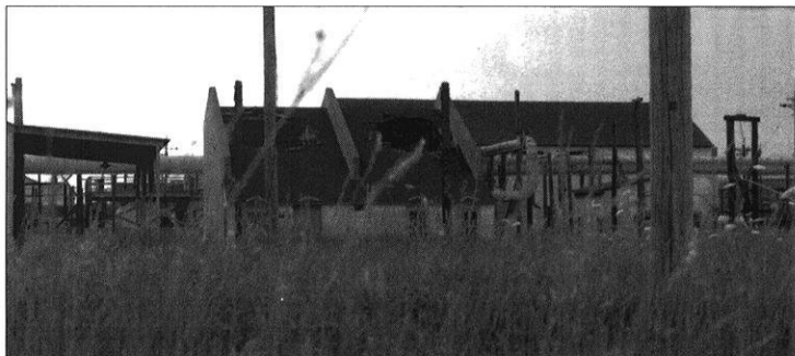
Holes punched in the roof allow space for equipment removal.
