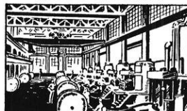
MAKING THE CABLE
