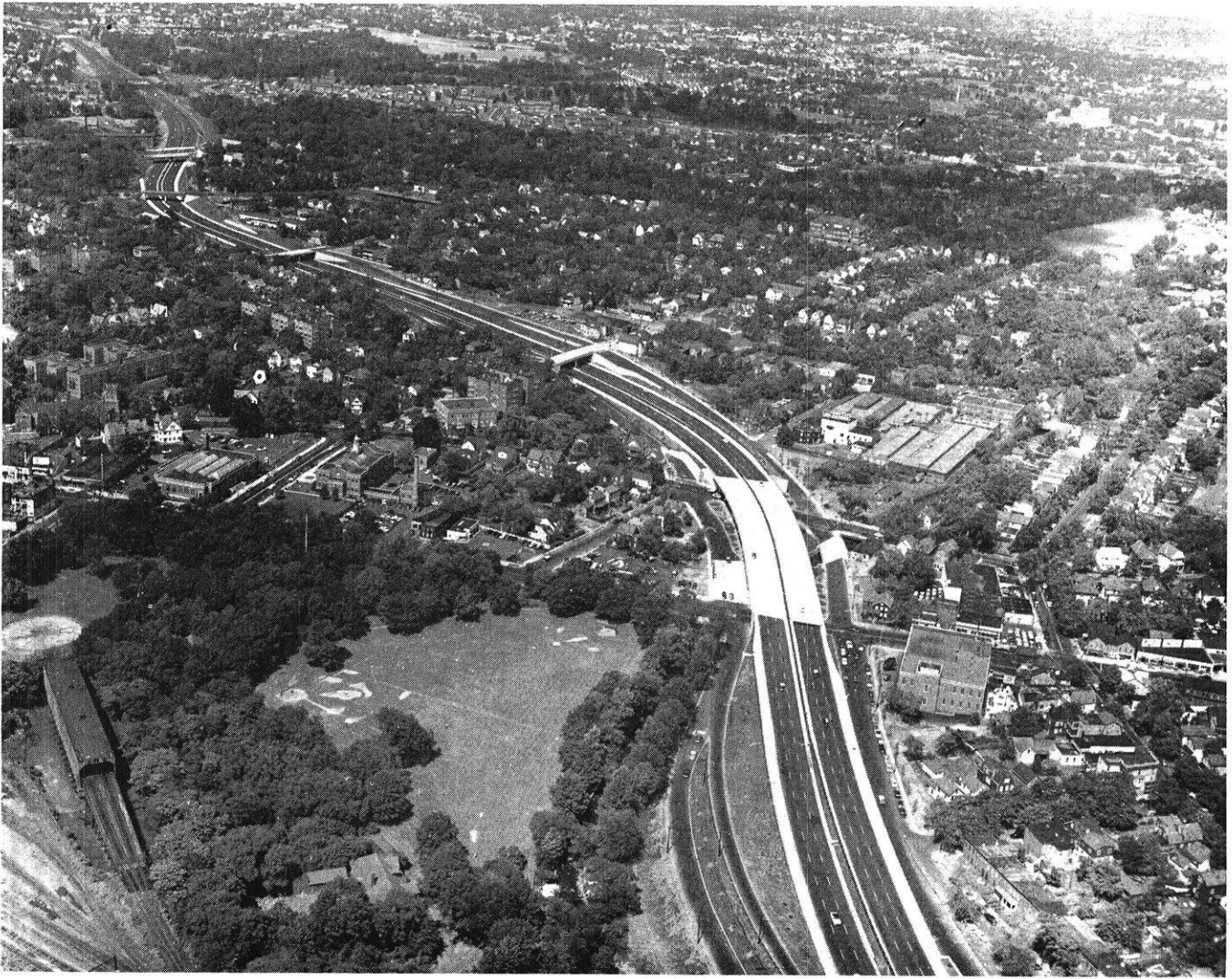
Garden-State Parkway. An excellent example of the problems met by the route surveyor.
