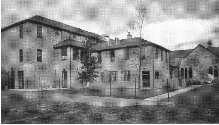
The Family Life Center before construction.
