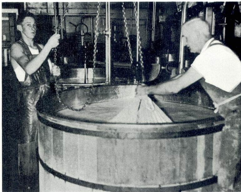
The inside of a cheese factory which shows curd being lifted from the vat to be drained and pressed into forms. Wisconsin makes one-half of the nation's cheese annually or about three pounds for every man, woman, and child in the United States.
