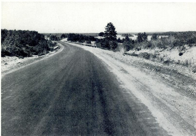
A typical dustless highway. During 1939, 14,297,235 gallons of bituminous material were applied to 1,885 miles of the state's highways to keep them free from dust.
