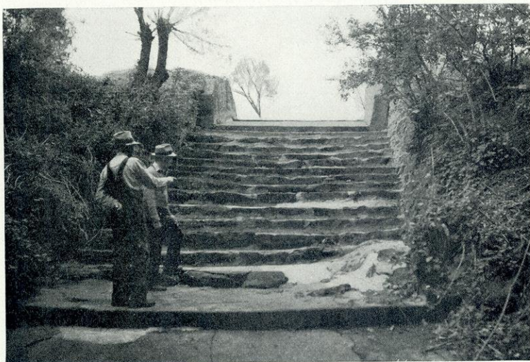
FLUME BUILT 30 YEARS AGO BY TREMPPEALEAU COUNTY FARMER. When a gully threatened to destroy a large part of his farm, this man used native rock to build this flume at the head of the gully and prevent it eating farther into his fields.
