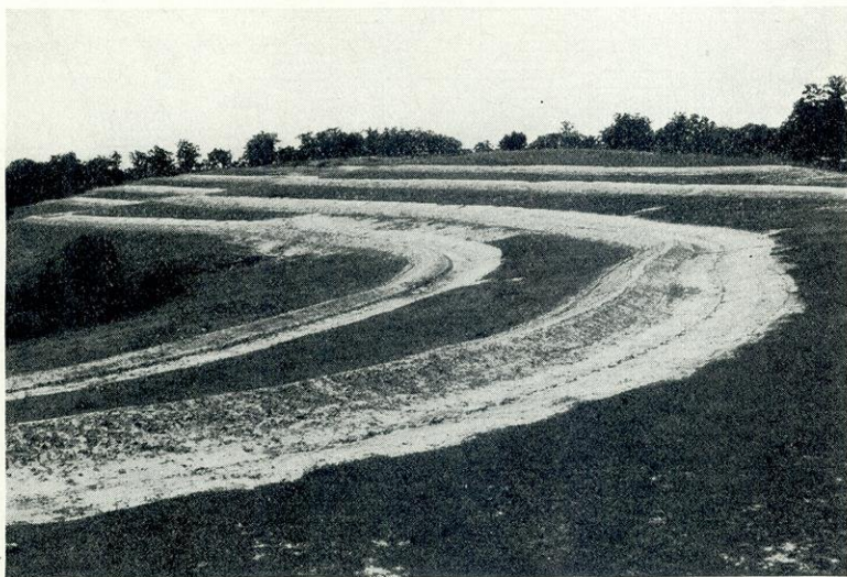
TERRACES ENABLE WATER TO "WALK—NOT RUN." A machine much like a road grader has been used on this field to throw up broad but shallow ditches at right angles to the slope of the land. These terrace ditches carry the water slowly to the sides of the field and then it runs down hill in prepared water courses that are resistant to the cutting action of water.
