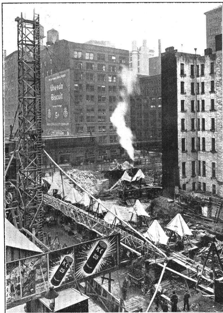
FIG. 3.—Caisson Construction at the Insurance Exchange Building, Chicago, Ill.
