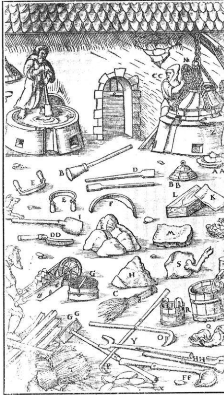
Preparation of Furnace Hearths in the Sixteenth Century. (Agricola.)
