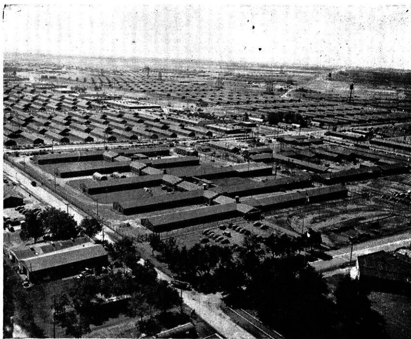
Air view of part of the Hanford Construction Camp. The Construction Administration Building is in the foreground. Picture is taken towards the southeast.
