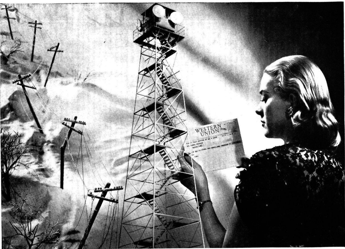
Radio relay towers, about 50 miles apart, will gradually replace thousands of miles of telegraph poles and wires.
