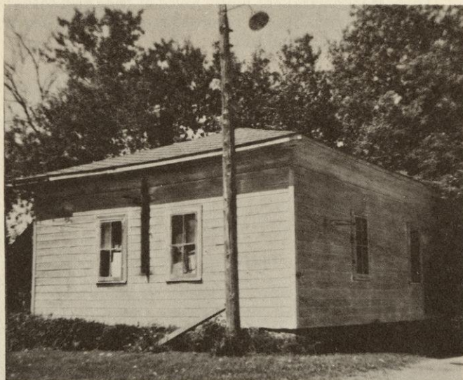
Building used for cheese making, still standing on the Otto Beilke farm, at 60th and Naugart Drive.
