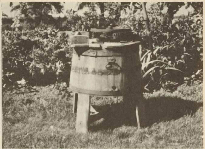
This washing machine was used by Mrs. Fred Scharbius in the early 1900's, and also by her daughter, Mrs. Arthur Utech. This early machine consisted of a paddle which worked as an agitator and was moved back and forth by the handle on the outside. The inside of the washer had a corrugated effect like a washboard.
