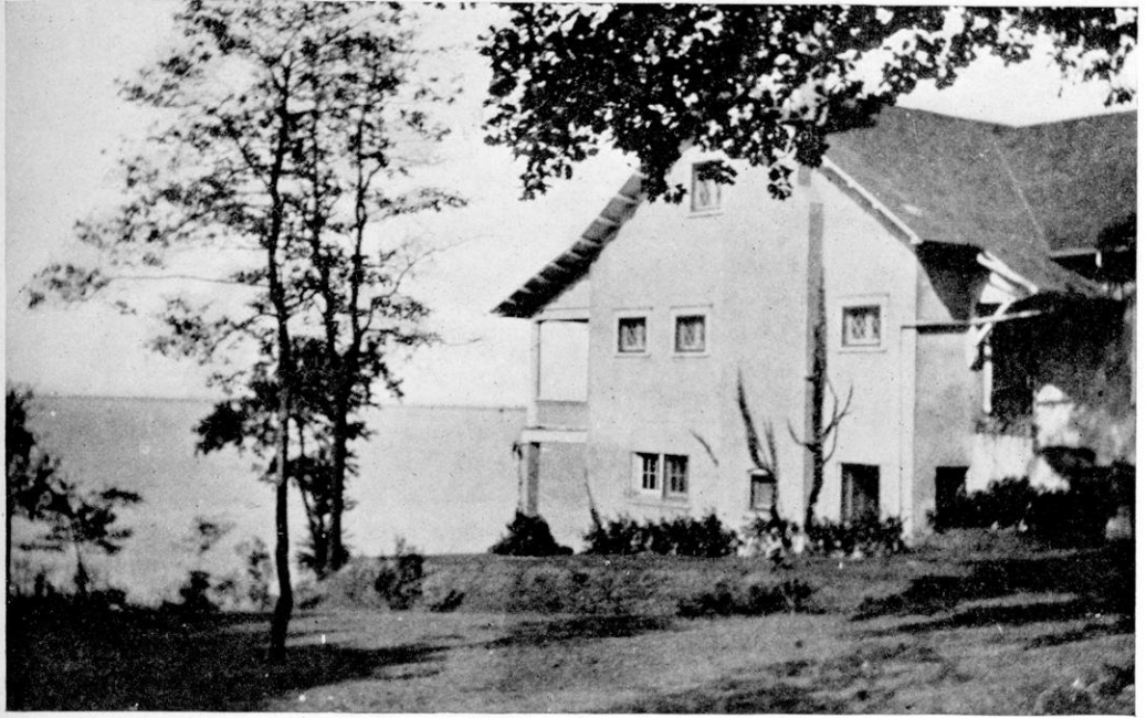
SHOWING SITUATION OF HOUSE ON THE BLUFF OF RARITAN BAY WITH WIDE PORCH RUNNING THE WIDTH OF THE HOUSE.
