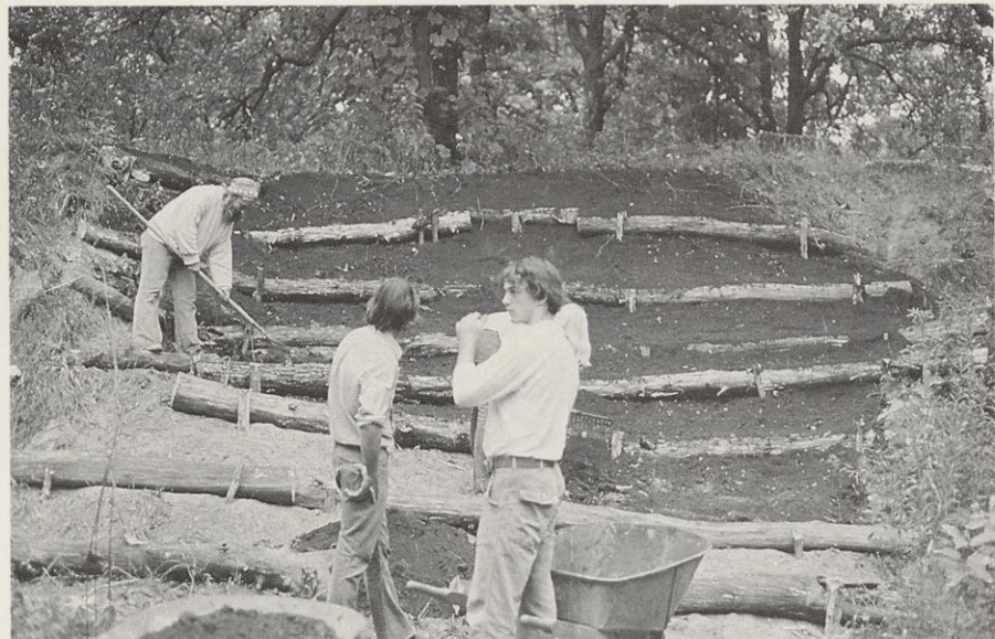
Volunteer workers terrace an eroded slope to control runoff.
