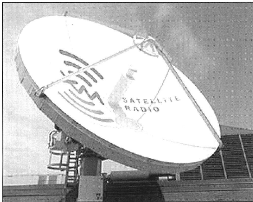
One of XM's two seven-meter uplink satellite dishes is located at the company's Washington D.C. headquarters.
