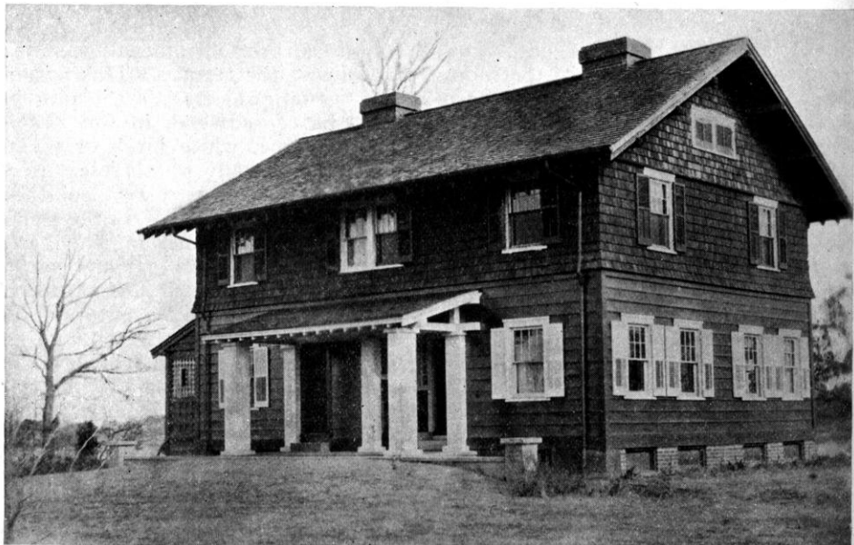
A HOUSE OF SEVEN FIREPLACES, BUILT AND OWNED BY MR. AND MRS. FRANK HUTCHINS
