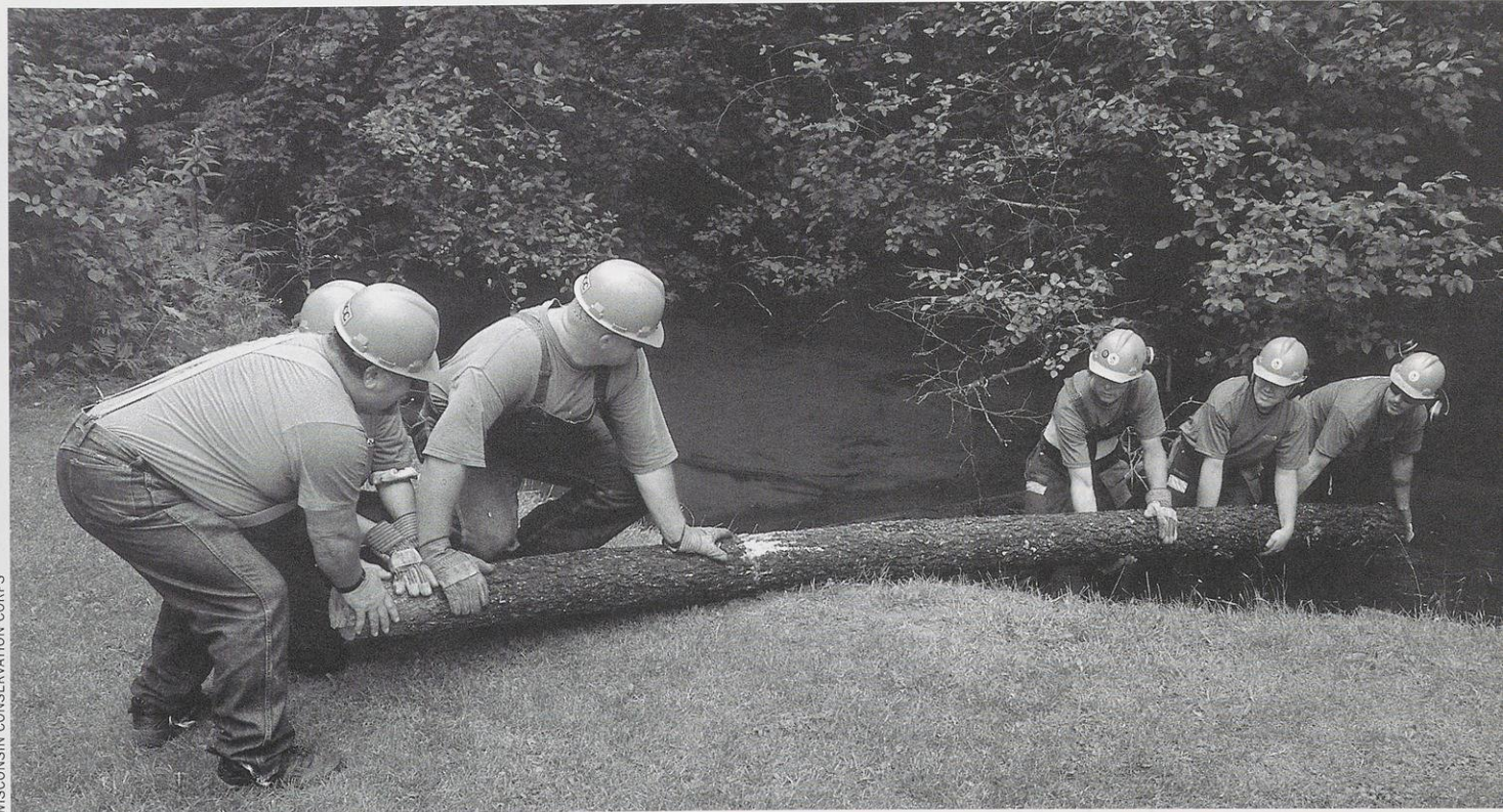
Crews install log structures in trout streams to increase water flow and provide shelter.
