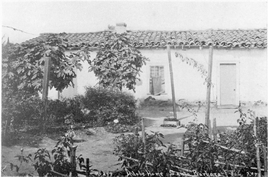
METHOD OF LAYING A ROOF WITH SMALL MISSION TILES. AN ADOBE BUILDING RE- QUIRES A MASSIVE ROOF.
