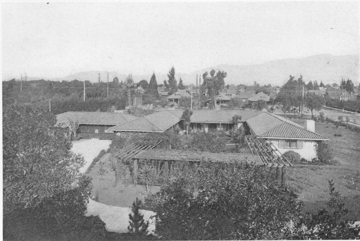
A WELL-LAID ROOF OF MODERN TILES: WATERTIGHT AND IM- PERVIOUS TO HEAT AND COLD.
