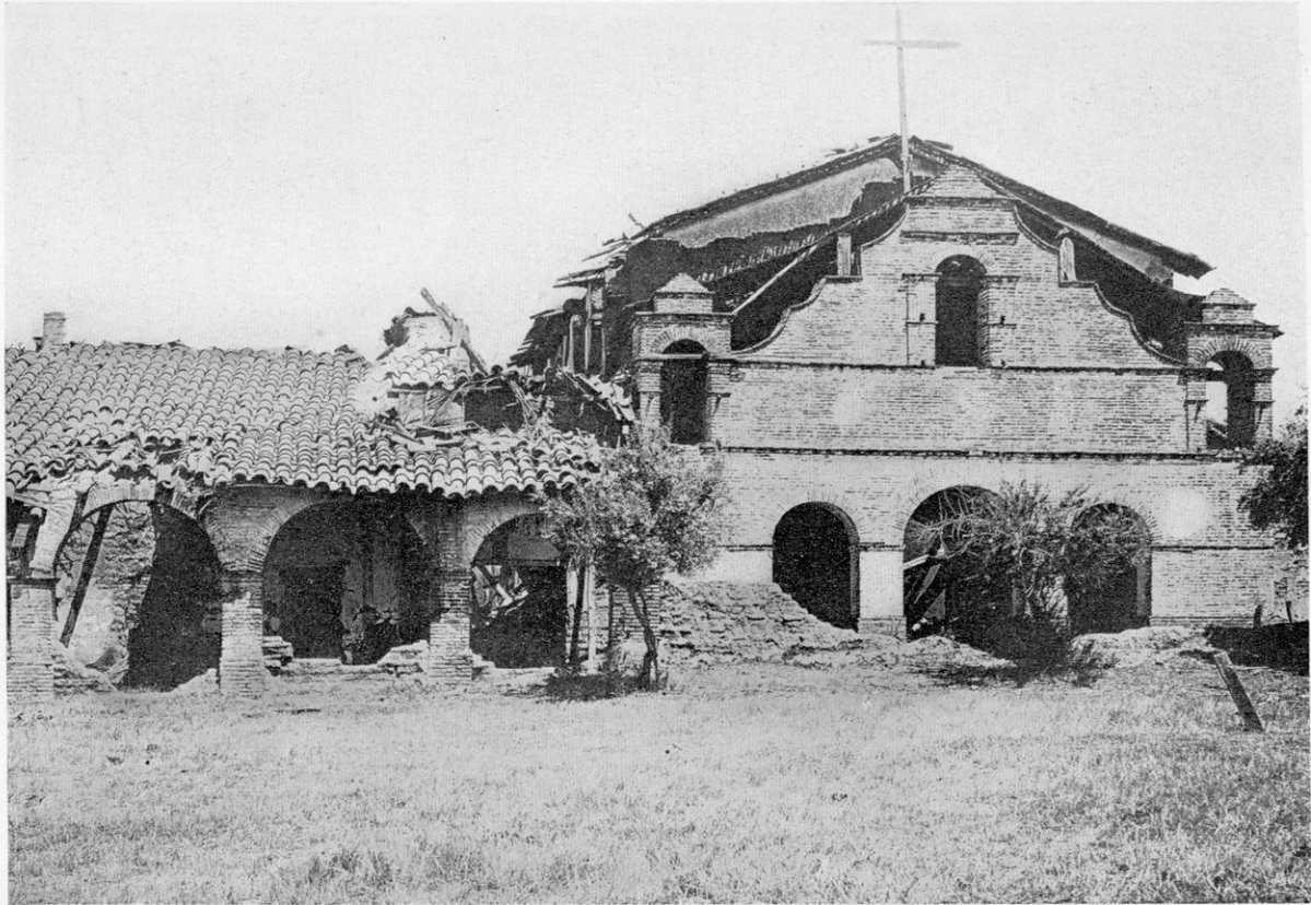
THE HEAVY OLD MISSION TILES WERE DESIGNED FOR BUILDINGS THAT WERE STRUCTURALLY MASSIVE.
