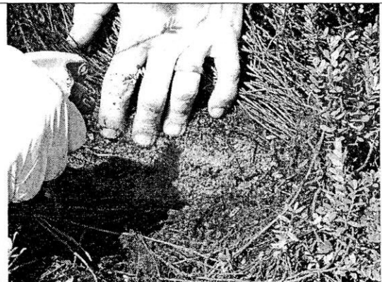
The membrane is watered into the soil to ensure good contact.
