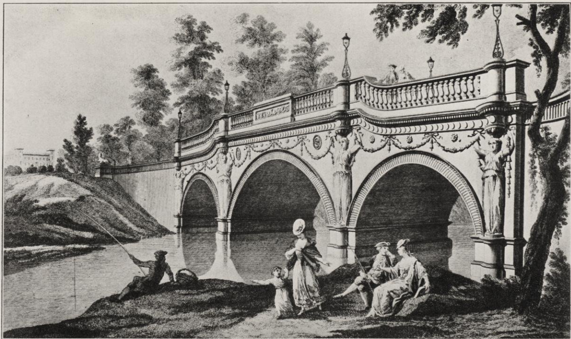
Design for a bridge from "The Works in Architecture of R. & J. Adam"
